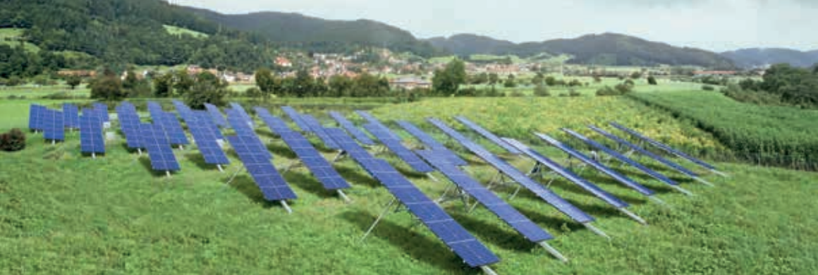
The Rheinau site. 28 compact and easy-to-install SunCarrier 22 tracking systems generate 135,000 kWh of electricity each year.
